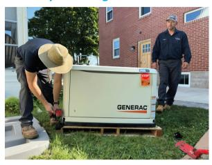
Our electricians carefully remove the generator from the pallet on to the platform.
