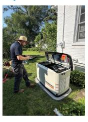
The generator is screwed down to the platform.
