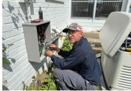
Generator Panel Installation: Our electricians will determine whether the generator panel can be installed inside or outside.
